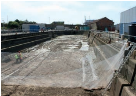
We used a subsea dock including a replica seabed
